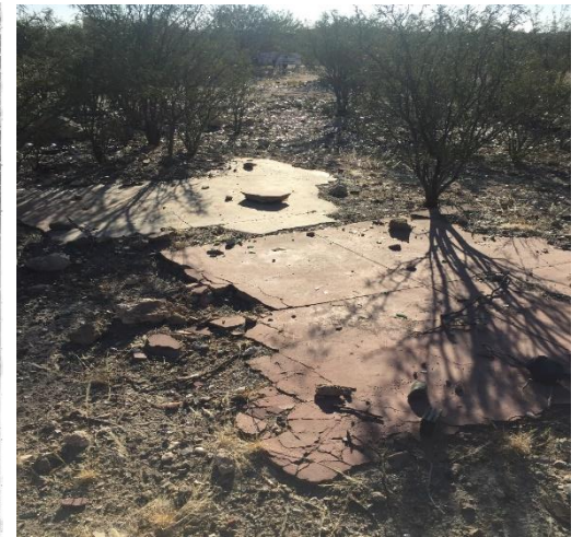
The foundations of one of the buildings that was removed from the Old Location.
