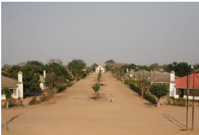
Chicualacuala, Main street. Down the street is the church. Behind, at the other end of the street is the railway station.
